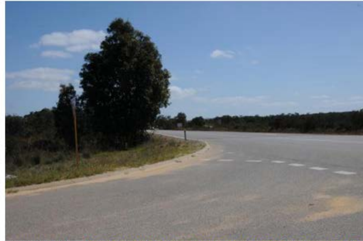
Finding 2.1 – Tree obscuring visibility to the south at the intersection
